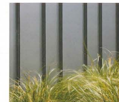
Varying the width of the tray is a design feature available with Eurostyle™ metal Cladding
