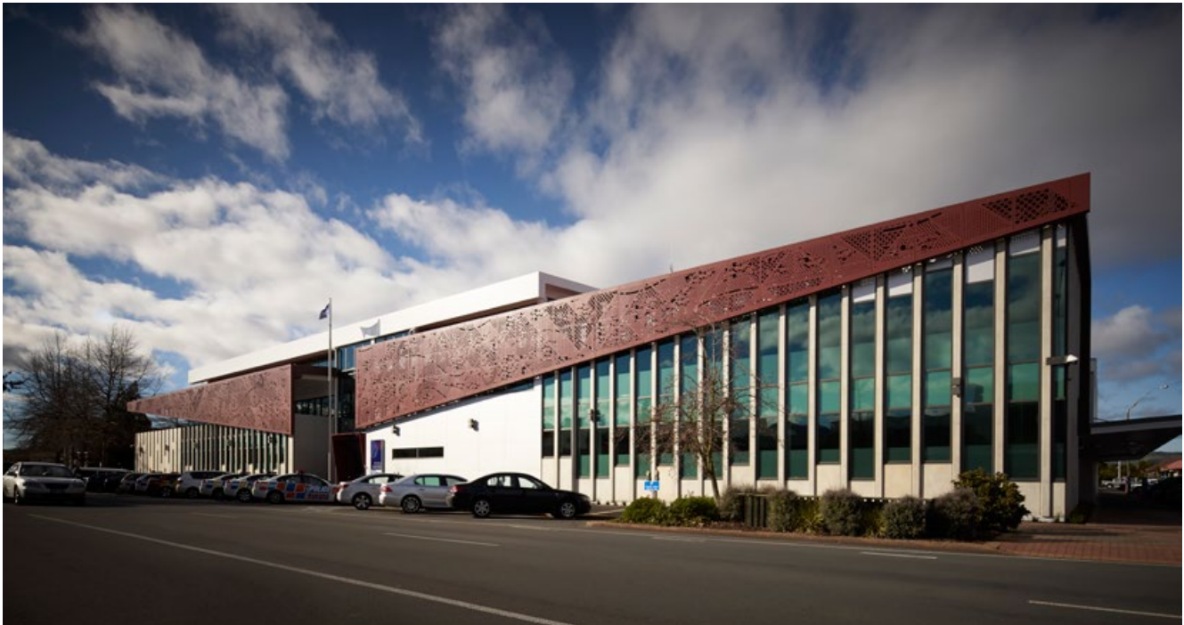
Referentially yours: Rotorua Police Station by Leuschke Group
