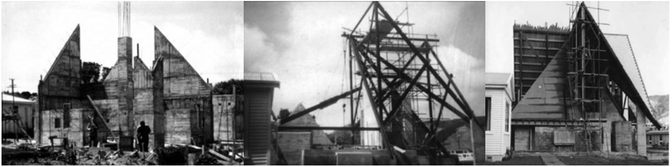
The Chapel under construction in 1960
