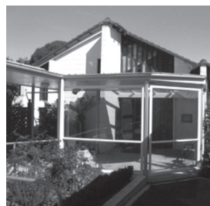
4 1964-65 Chapel of the Good Shepherd Waiapu House, Danvers Street Havelock North
